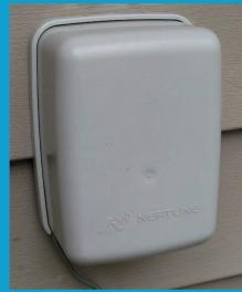
In most cases, a transmitter is mounted on the outside of the building for wireless transmitting. It replaces the reader touchpad when the old meter is removed.
